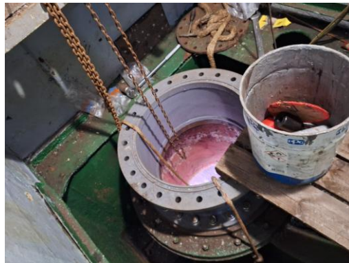
Flange adapter installed
