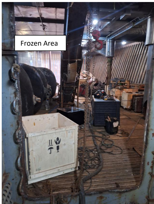
Works done on sonar room to install the hull unit (upper deck)
